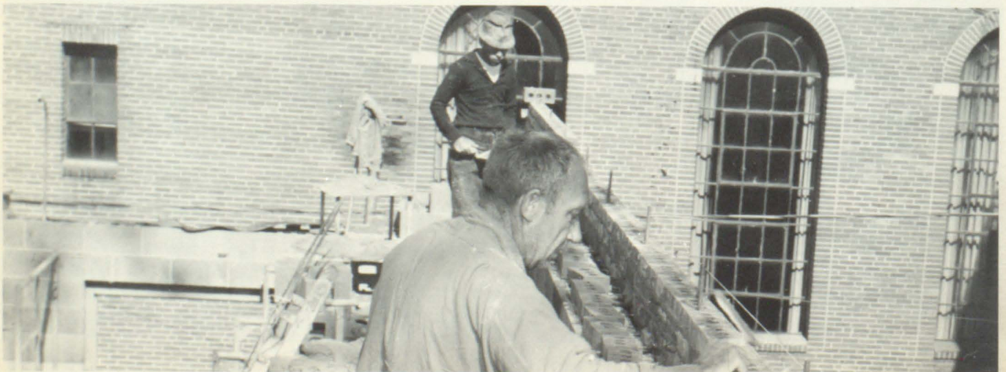
Construction of Our New Lunchroom In Progress "When do we eat. . . . in our New Lunchroom?"
