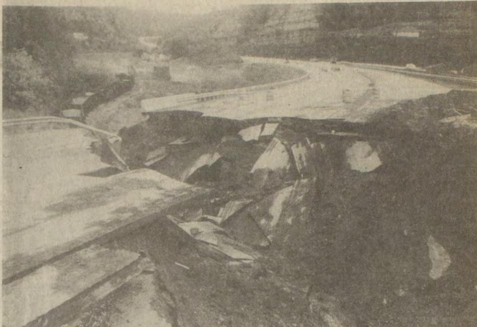
FLOYD'S NEWEST highway was split by this ragged trench early Sunday morning, when a corrugated iron tunnel, built to accommodate a railroad track up Bucks Branch, suddenly collapsed. Two cars plunged into the rift but both drivers escaped serious injury. The \$600,000 culvert, which has had a tendency to sag almost since the highway was constructed six years ago, was previously braced once and was scheduled to be shored up again next month. Now it is to be replaced by a bridge.
