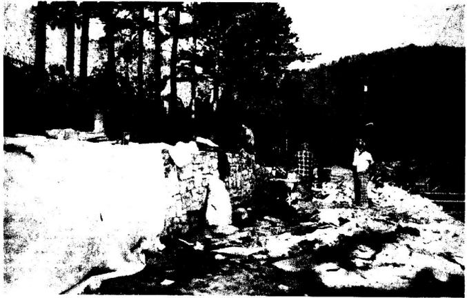
Although the dredging project planned for Brandy Keg Cove awaits drawdown of Dewey Lake by the U. S. Army Corps of Engineers, the P & N Construction Co., of Lexington, has begun other work as part of the planned renovation of the Jenny Wiley boat dock facility which is located in the cove. Shown under construction here is a cut-stone retaining wall bordering an access road to houseboat moorings.
